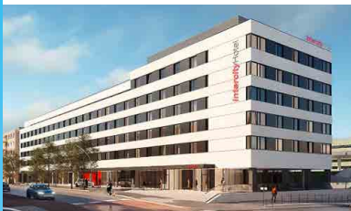
IntercityHotel Investment financing Graz/Austria Arranger and lender: UniCredit Bank Austria AG February 2021
